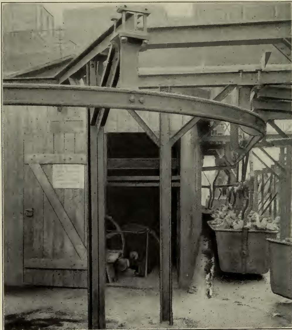
FIG. 24. ELECTRIC TELPHERAGE FOR SURFACE TRANSPORT AT A MINE.
